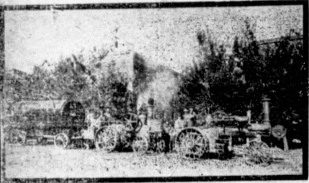
One of the two big boilers that were taken to the Cullen Mine, on a wagon especially built for the purpose and drawn by two engines.
