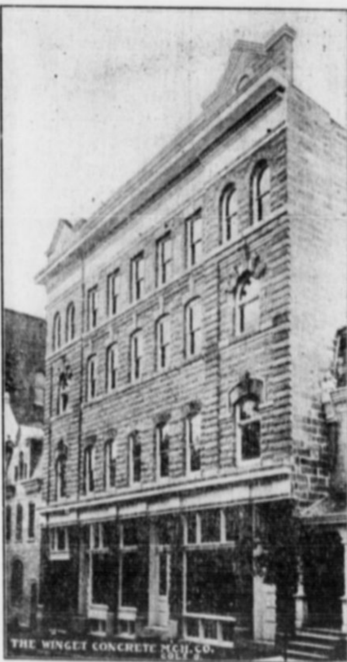
Store room and apartment block. Especially suitable because the first story is an eighteen-inch wall, showing the practicality of the Winget concrete block.
