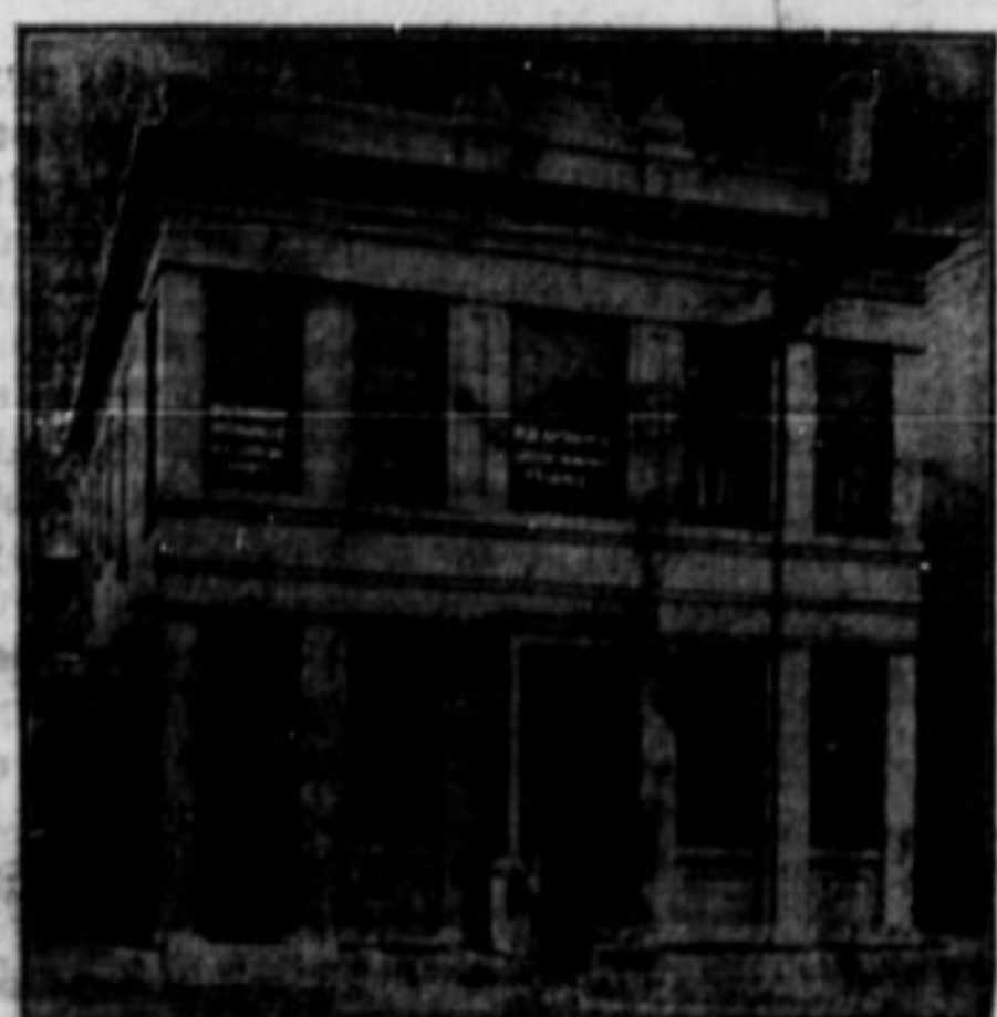
Postoffice Building, Bucyrus, O. Built of hollow concrete blocks, plain face, made on the Winget Machine.
