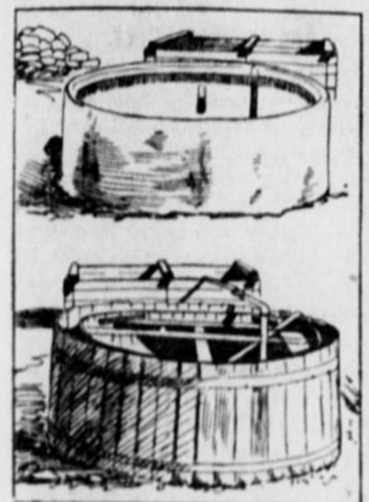
STAVE MOLD FOR CEMENT TROUGH AND THE TROUGH COMPLETED.
