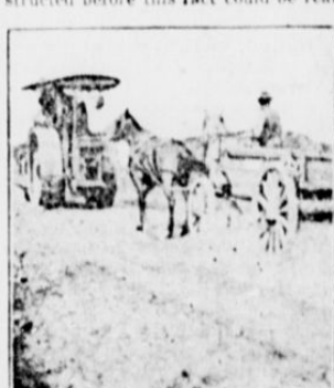
Constructing Road Sections for Impact Tests.
