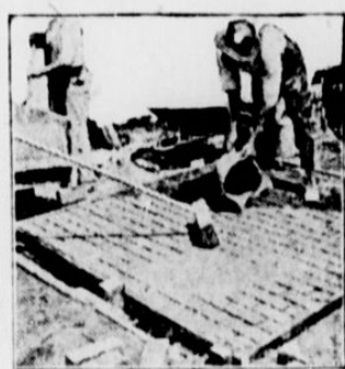
Laying Brick Pavement.
