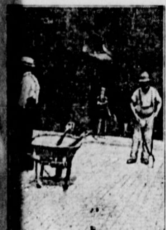
White blocks Laid and Rammed — Maintenance Cost of This Kind of Pavement is Less Than That of Any Other Kind.
