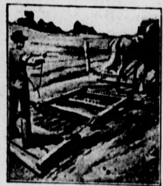
The Spiked Forward Part of the Drag Loosens the Road Soil, and the Following Rear Portion Packs It to a Smooth Surface, Thus Finishing the Surface in One Operation.
