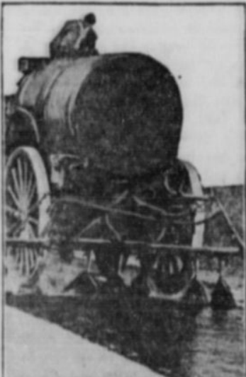
Treating the Surface of a Macadam Road With Bituminous Material.
