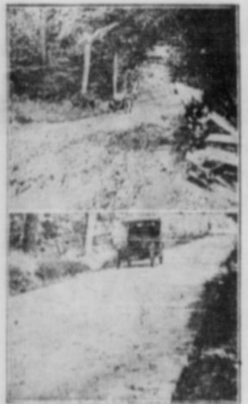
The Brotherton-Berlin Road in Pennsylvania, Showing How It Appeared Before and After It Was Improved by a Concrete Road-Bed.
