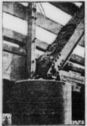
A Dangerous Bridge—This Rusting Could Have Been Prevented by Painting.
